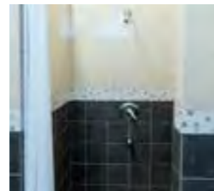
REST ROOM & SHOWER
